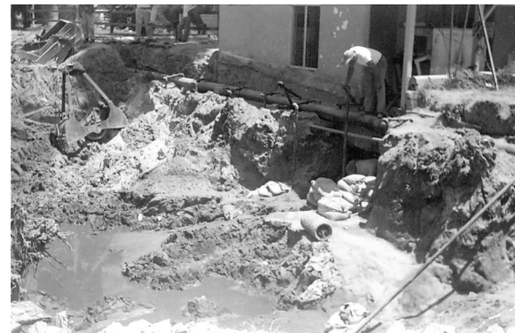
The widening of Indian Avenue in downtown Palm Springs (now North Indian Canyon Drive) at the Tahquitz intersection, shown here in various stages, began in 1953. The road's expansion covered the Hot Mineral Spring, so a holding tank, or collection ring, was built to maintain access to the water.
