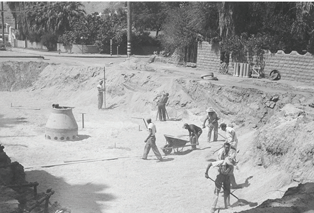
The widening of Indian Avenue in downtown Palm Springs (now North Indian Canyon Drive) at the Tahquitz intersection, shown here in various stages, began in 1953. The road's expansion covered the Hot Mineral Spring, so a holding tank, or collection ring, was built to maintain access to the water.
